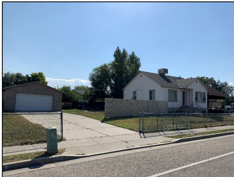
Subject Property – east façade and driveway 2 on California Ave
