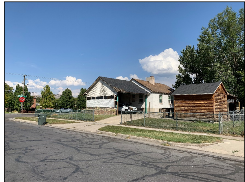
Subject Property – rear facade
